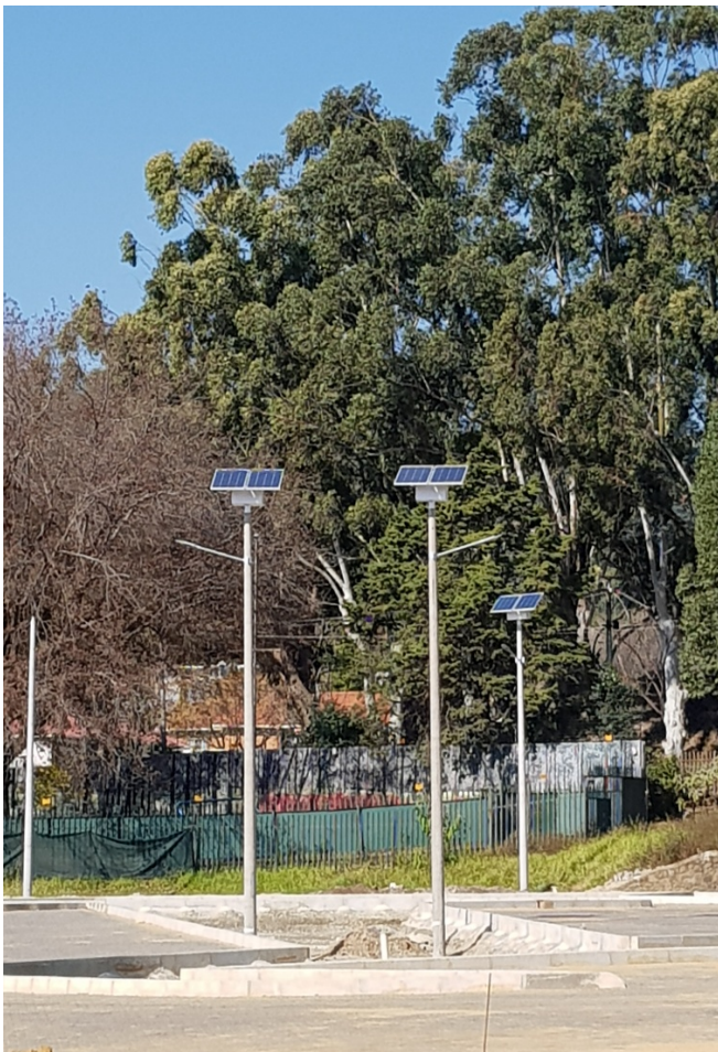
Above model is a 60w on an 8 meter surface Concrete pole
